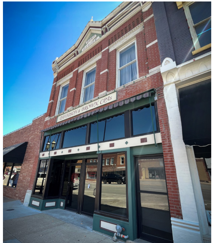
Proper proportion ensures that the elements of the sign are balanced with the building.
